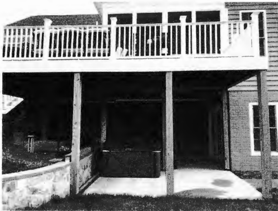
Hot Tub under back desk on a 3+ inch concrete slab
