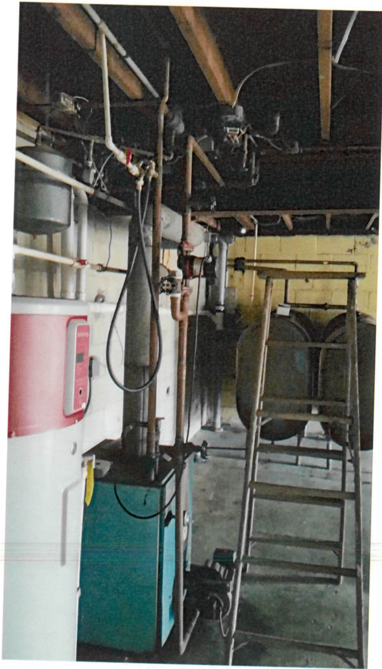
Basement parcel 1, septic line behind oil tank.
