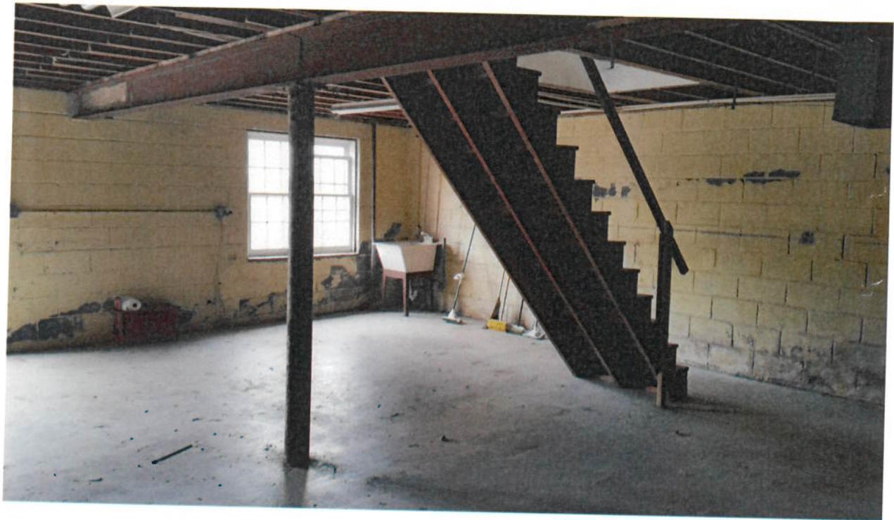
Basement parcel 1, utility sink into slab.
