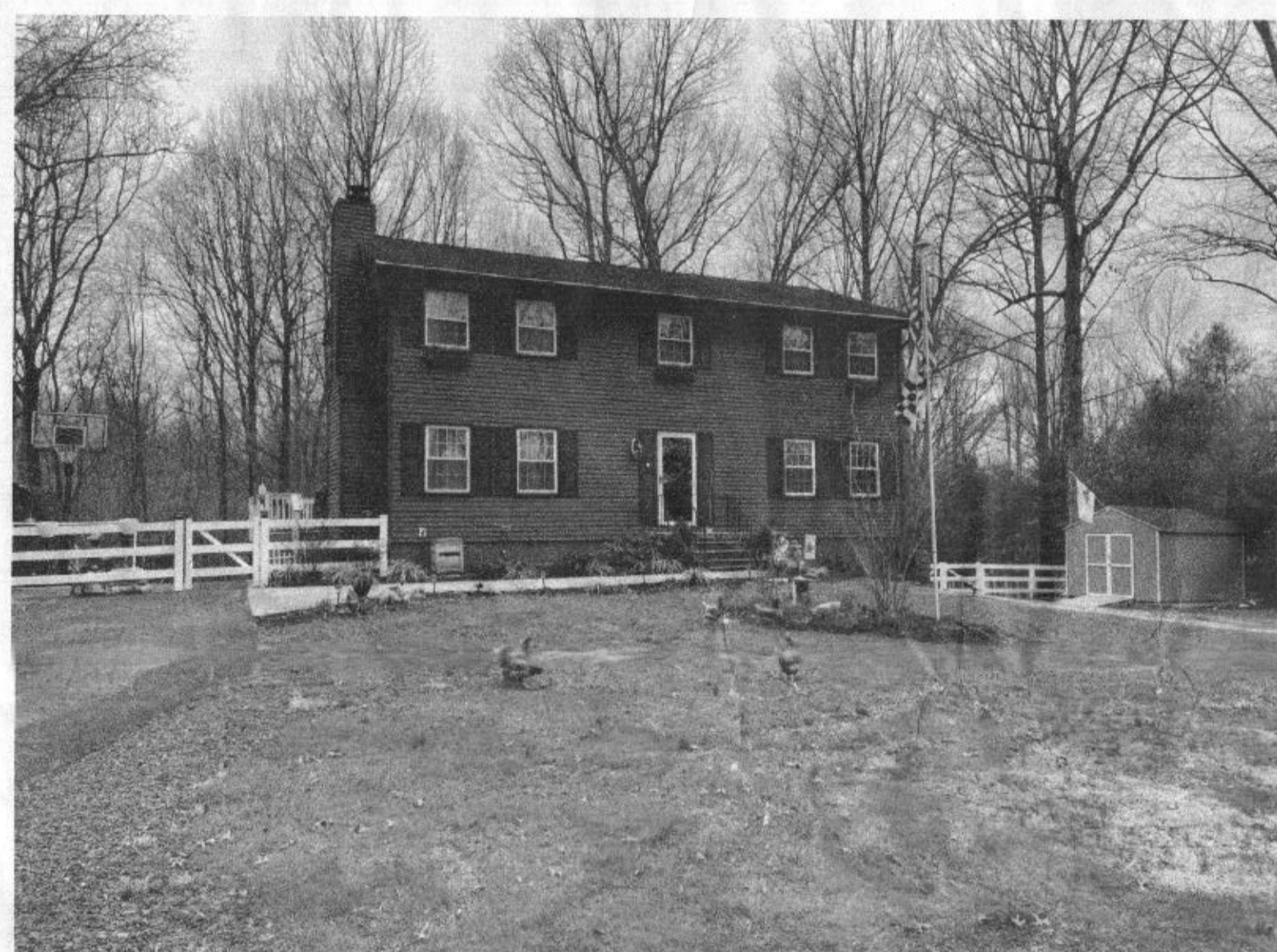
PICTURE: EXISTING CONDITIONS
