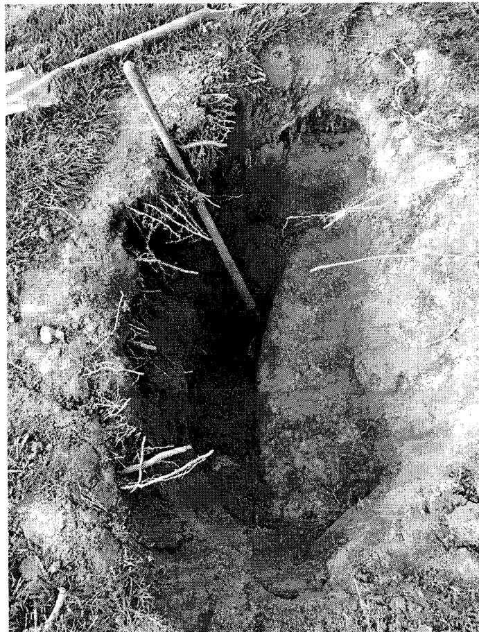
Exposed concrete top of dry well
