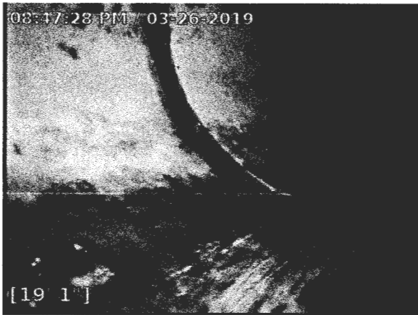
3/26/2019 8:47:29 PM Shows a right bend in the PVC front line.
