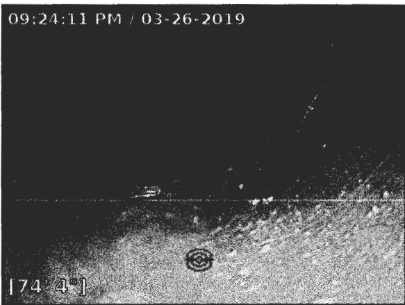
3/26/2019 9:24:12 PM The camera could not be advanced past this point in drainfield line B due to multiple bends and length of the drainfield line. The camera was advanced in drainfield line B from this point back towards the distribution box.
