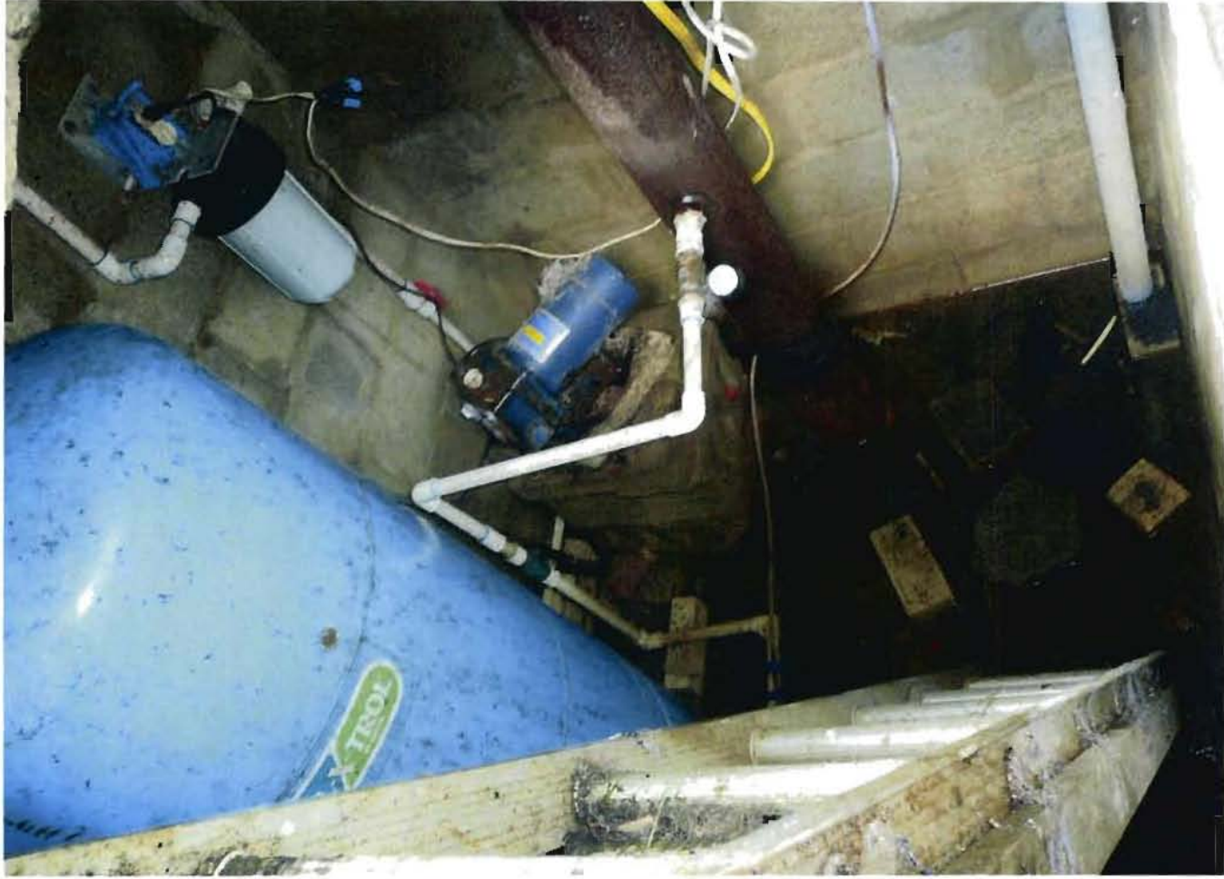
Inside view of shared well pit.
