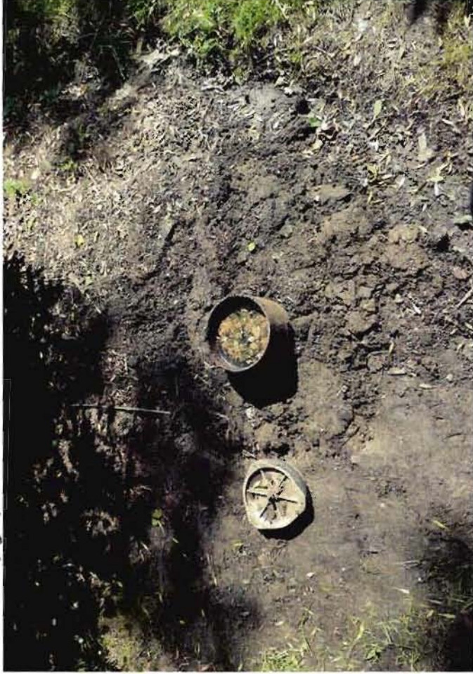
SEPTIC TANK CLEANOUT
