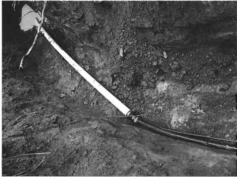
Images from well line installation on 12/24/16 sent by Fogle's Well Drilling on 1/10/17 (HCHD did not inspect well line)
