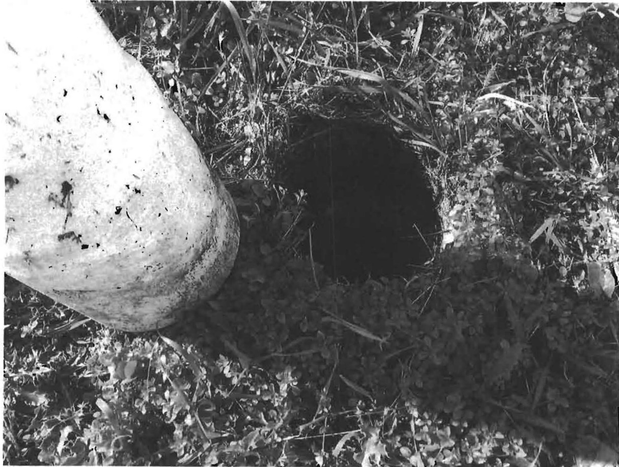
Well Casing - Top portion of well casing was removeable.
